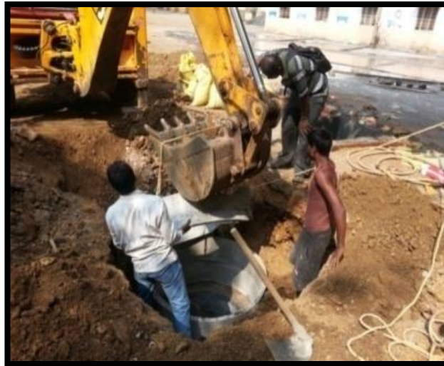
Construction of RWH Scheme
